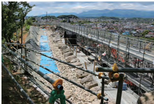
▲復旧作業が進む本丸北面の石垣
