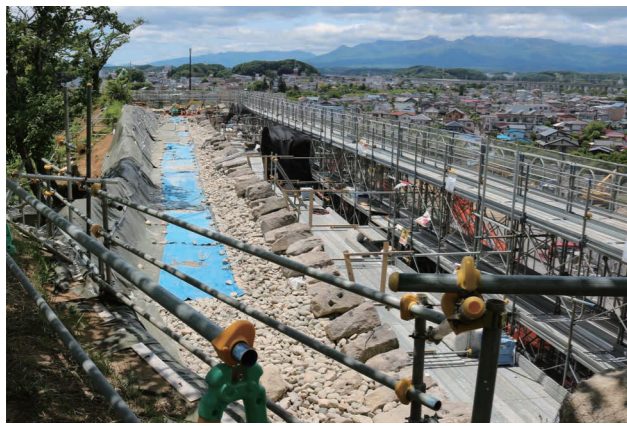
▲復旧作業が進む本丸北面の石垣
